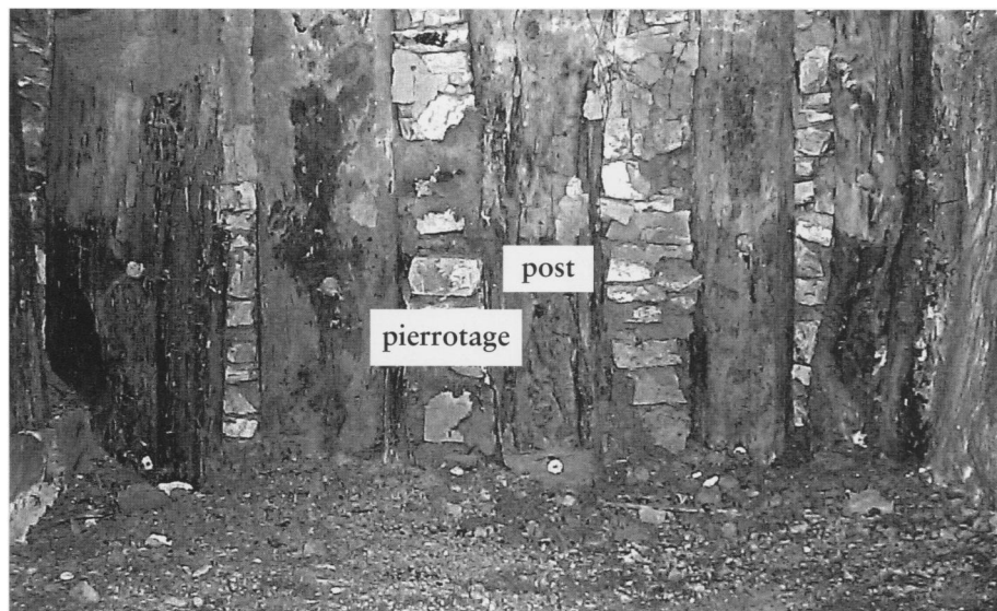
Fig. 2. Posts-in-ground construction viewed from the cellar of the Amoureux house, Ste. Genevieve, Missouri.
